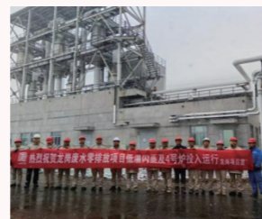
Successful commissioning of the Xuchang Longgang Project
